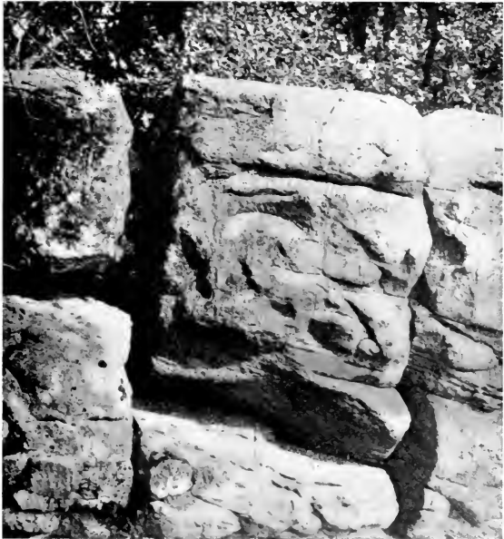
FIG. 13.—St. Peter sandstone, Iowa. Effects of joints and bedding planes on weathering. From Iowa Geological Survey.
